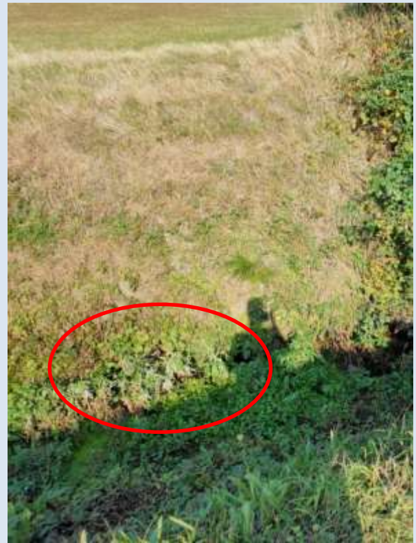
Confirmation of presence of water burrows previously identified in 2019 (ref WV-RCH1)
